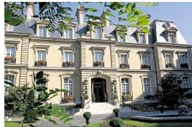
The hotel's exterior
